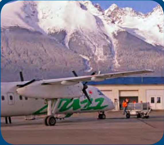
Upgrades to Smithers Regional Airport are important to expanding both tourism and mining opportunities in the Bulkley Valley
